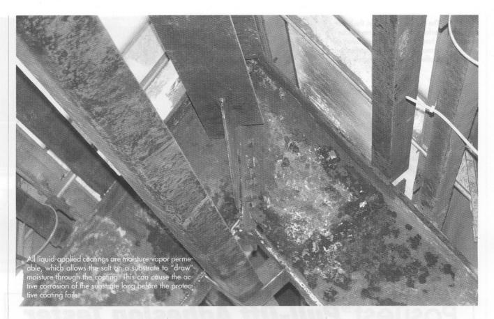
forming insoluble salts, thereby limiting salts from causing or increasing the corrosivity of the immediate environment. The widespread use of lead-based paints gave us a sense of security but the legislated ban of such products requires reevaluation of surface preparation requirements. Also, as new "high performance" coatings are developed, film thickness is decreasing. The thinner coatings get, the more critical soluble salts become.
